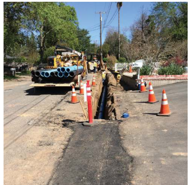
Rosa Vista Main Replacement Project.
