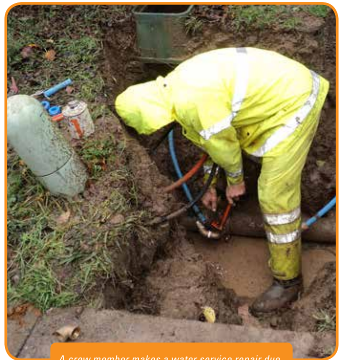
A crew member makes a water service repair due to a leak in the system.
